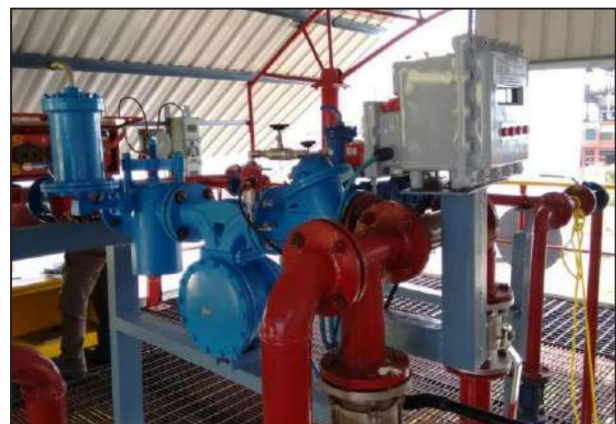
3" Meter with Electronic Configuration
