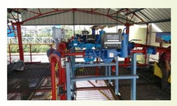
Vermont has wide range of Mechanical & Electronic Meter options ranging from 1" to 8". Our Flow Meters can be fitted with Mechanical Counters and Preset Valves or Electronic Preset Counter with digital counter valves. Both these counter versions are well suited for multiple applications such as: Batching and Blending operations in Lube Oil, Chemicals, Ethanol and Barrel filling.
